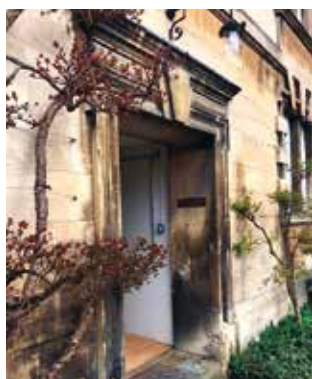
Entrance to V staircase
